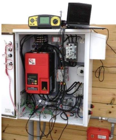
The figure above shows the Boxer, QFE Motor Controller and Metrel Power Meter
